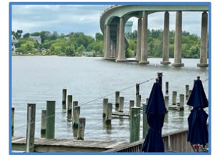
View from Severn Inn
