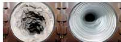
Dryer Vent Cleaning Before & After
